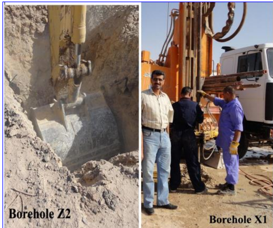
Figure 1-8: Methods of drilling the borehole in the study area. Trench method (left); rotary drilling (right).
